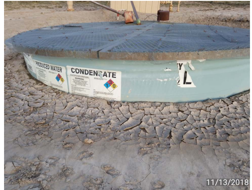
Photo 2. Tank capacity label is mostly missing.
