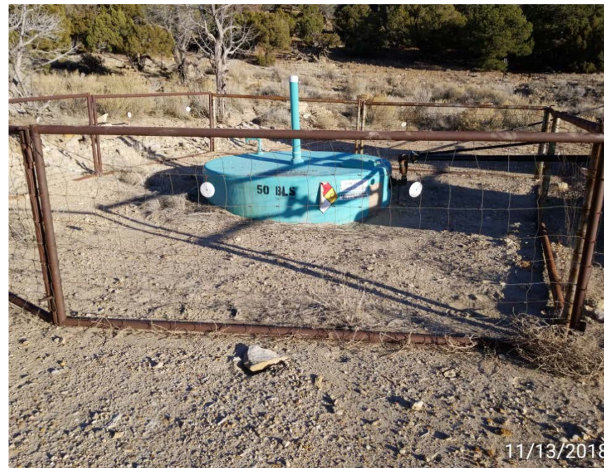
Photo 2. Tank with insufficient berm
