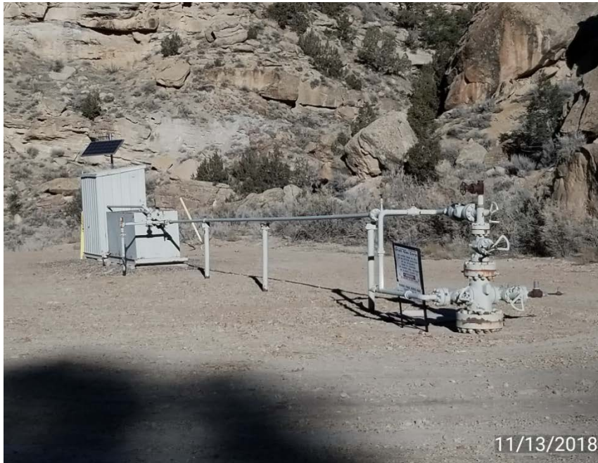
Photo 1. Location looking west
