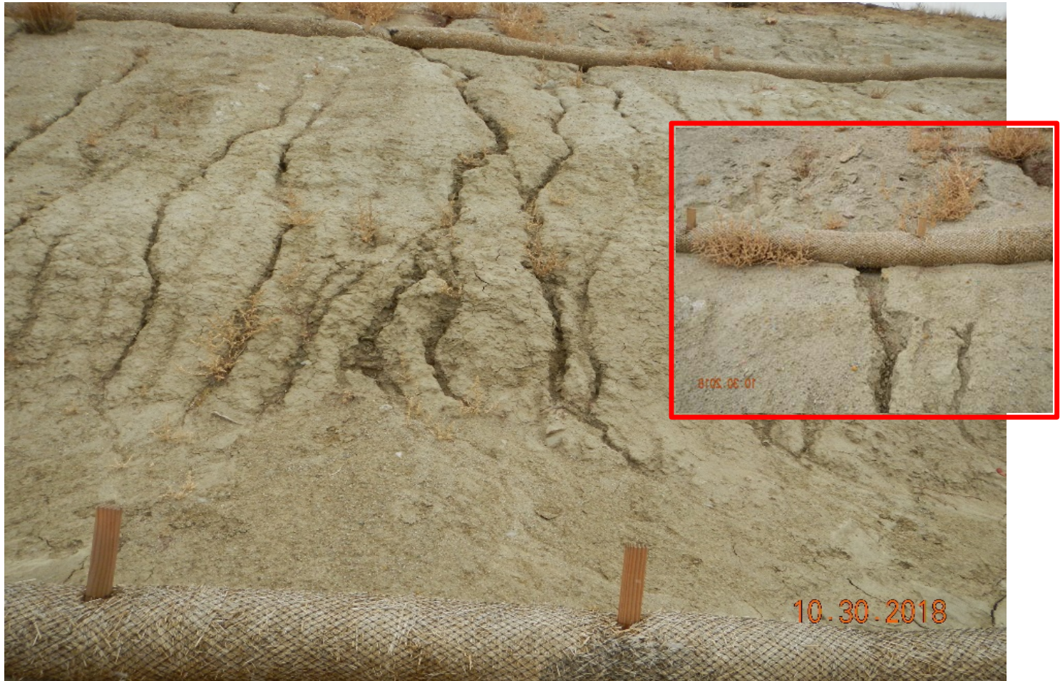
Photo#2: View of erosion on East Cut slope.
