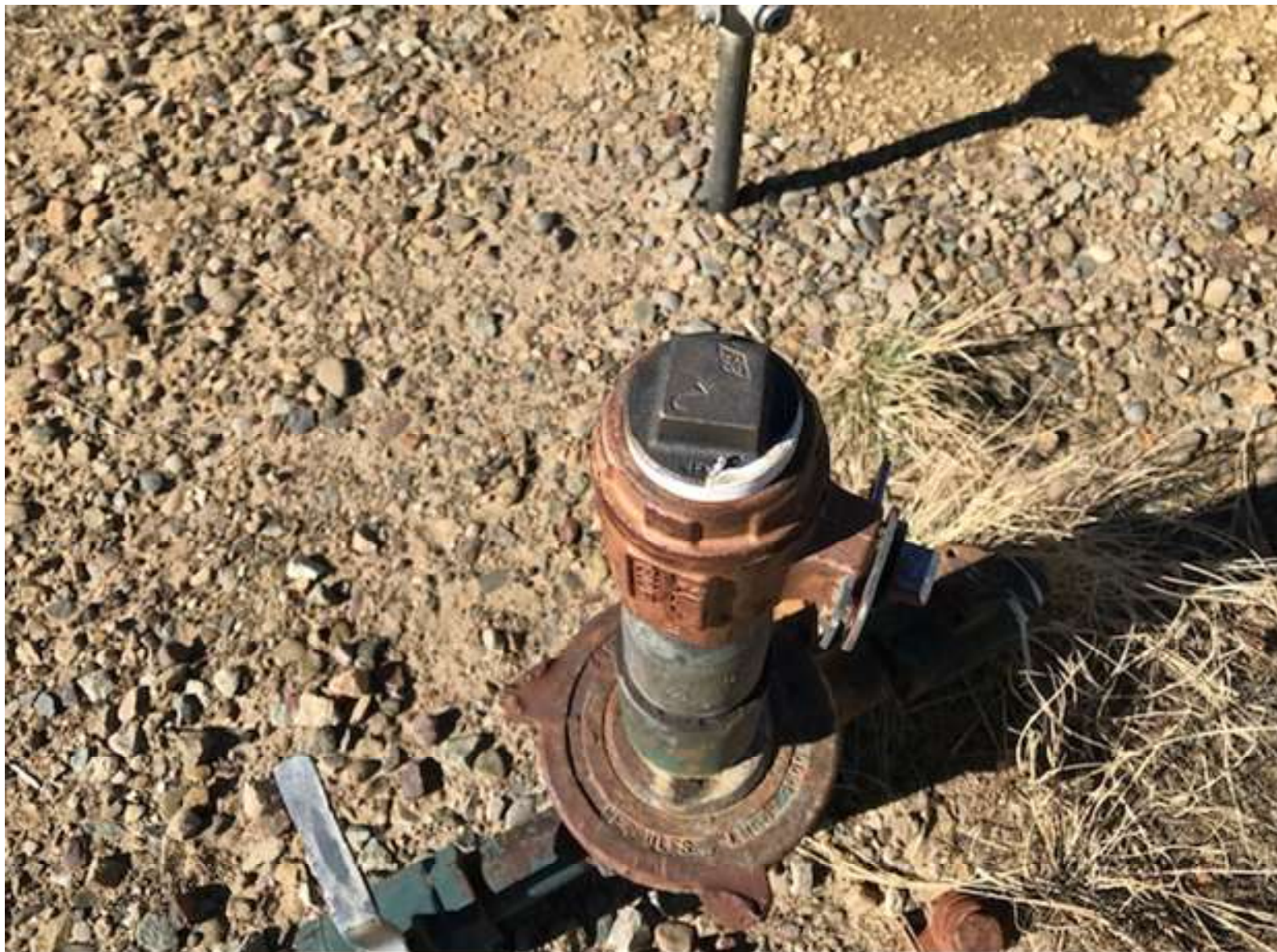
INSTALLED BULL PLUGS ON THE RISERS.
