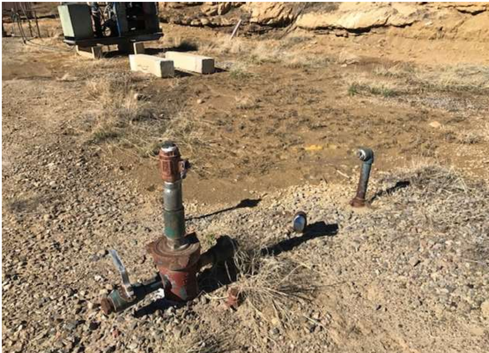
INSTALLED BULL PLUGS ON THE RISERS.
