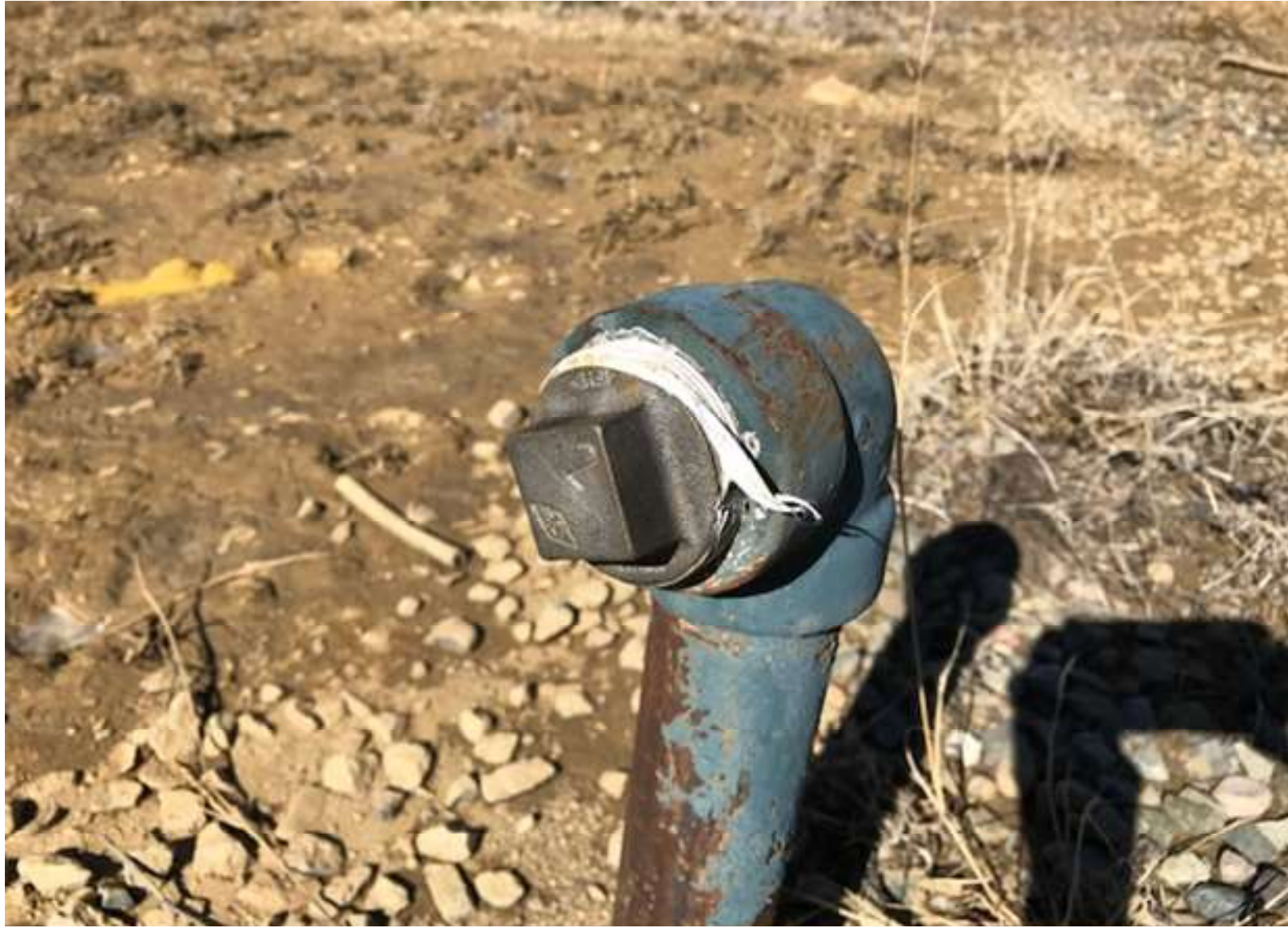
INSTALLED BULL PLUGS ON THE RISERS.
