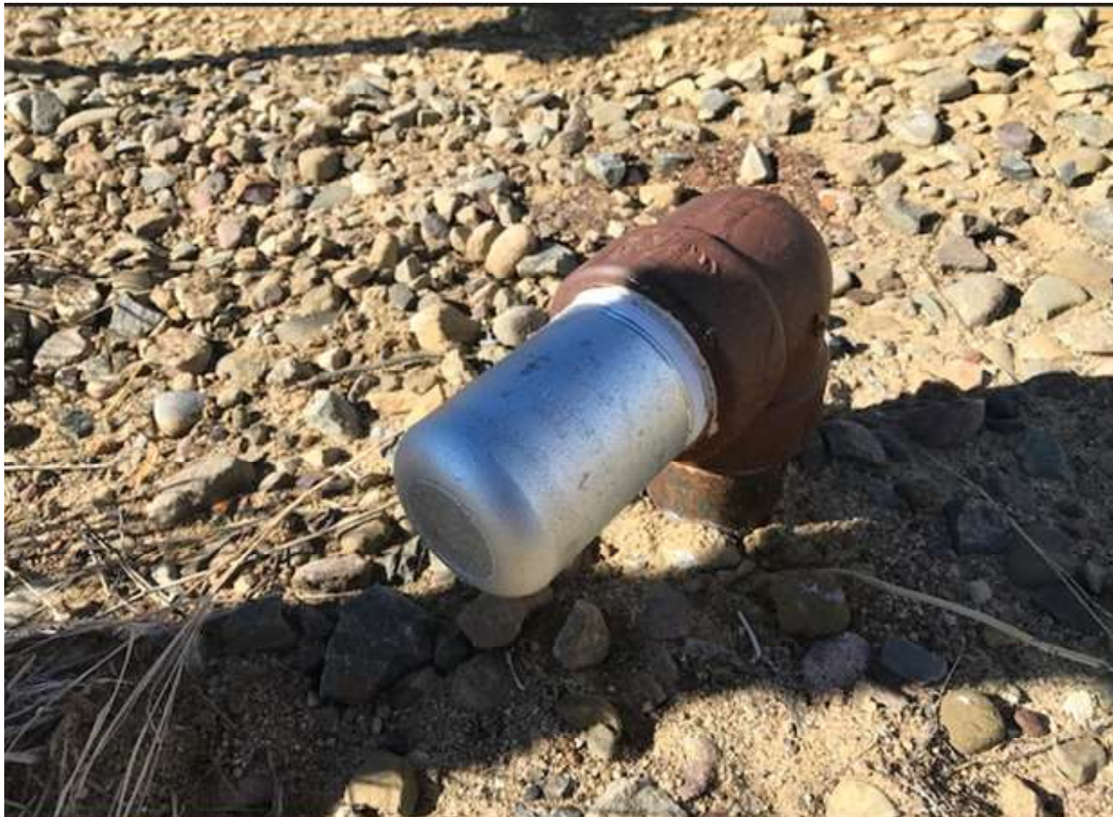
INSTALLED BULL PLUGS ON THE RISERS.
