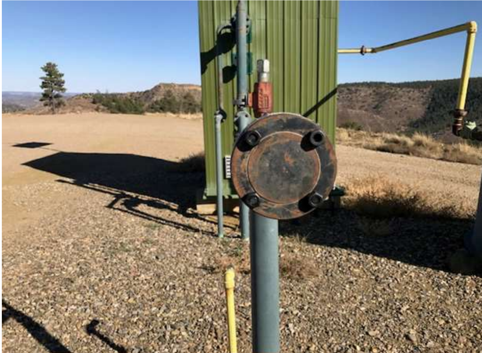
INSTALLED BULL PLUGS ON THE RISERS.
