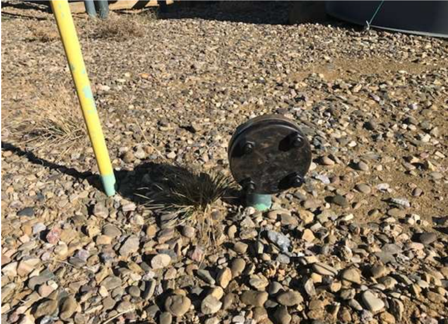
INSTALLED BULL PLUGS ON THE RISERS.
