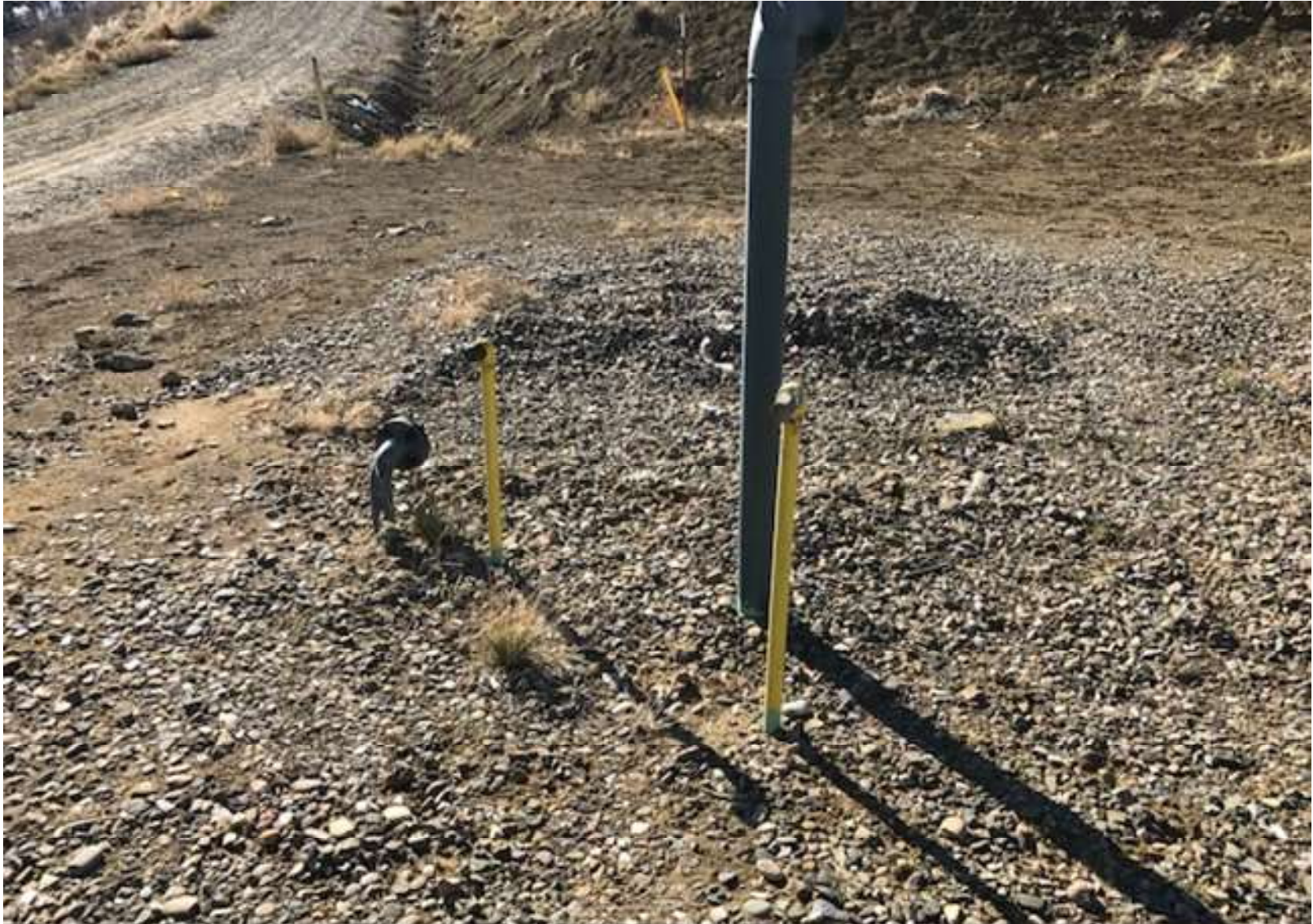
INSTALLED BULL PLUGS ON THE RISERS.
