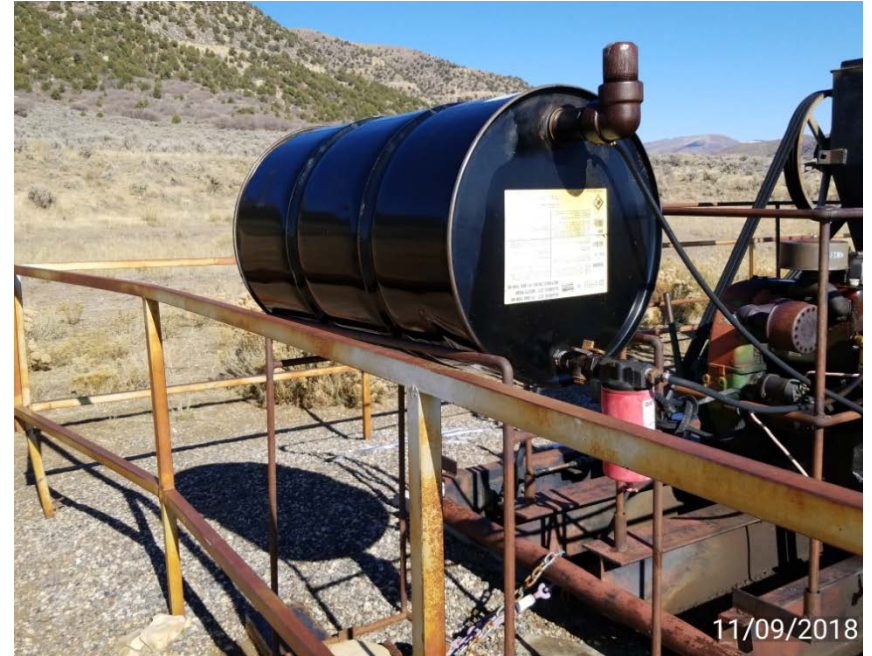
Photo 4. Container without secondary containment.
