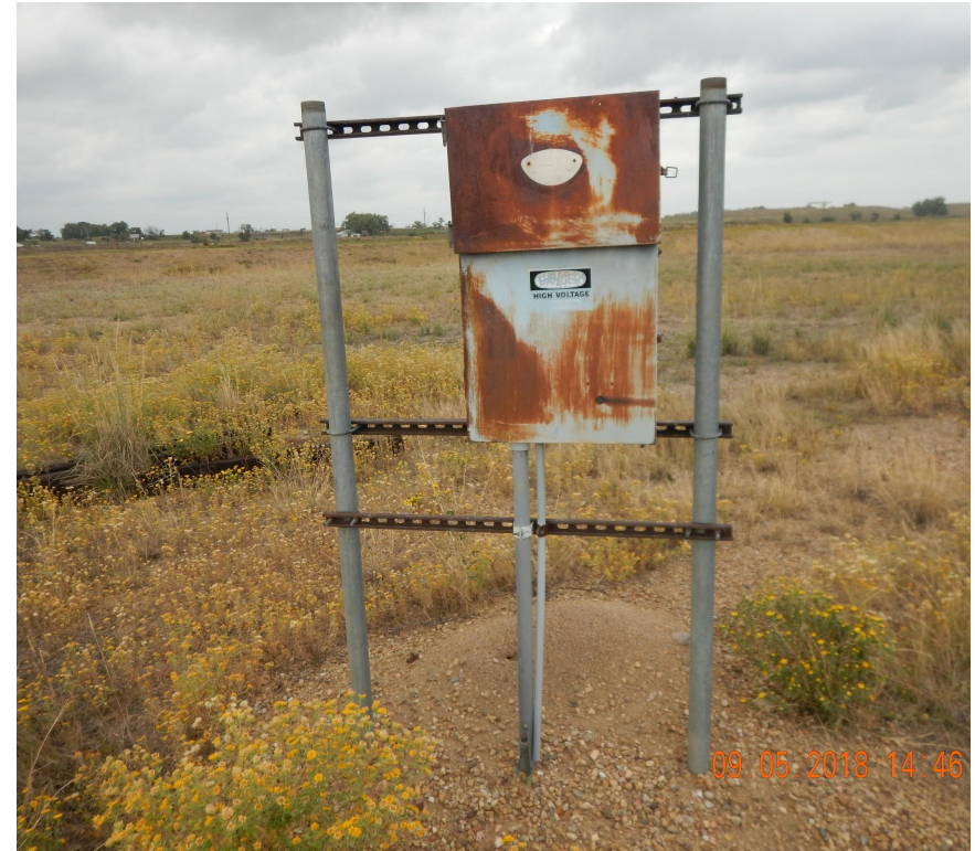
Photo 2. Photo taken from the location on September 5, 2018. Photo illustrates the Operator failed to remove equipment after previous corrective actions were issued.
