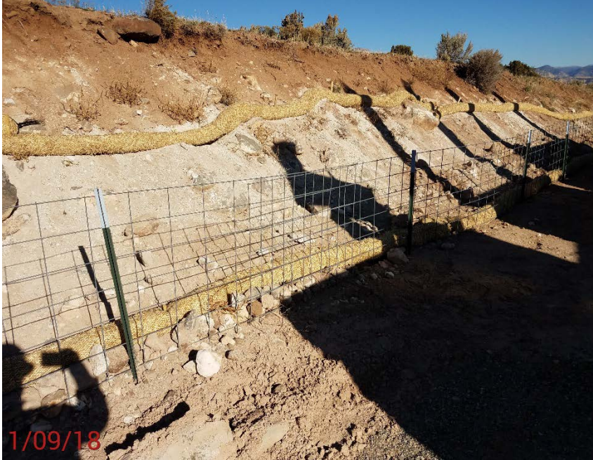
Location Photo #3, Waddles added behind separator to address storm water issue.
