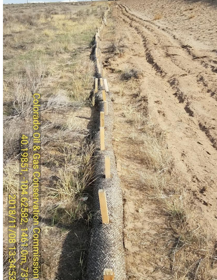
Photo 6 Waddles and Ditch on North Side of Location
