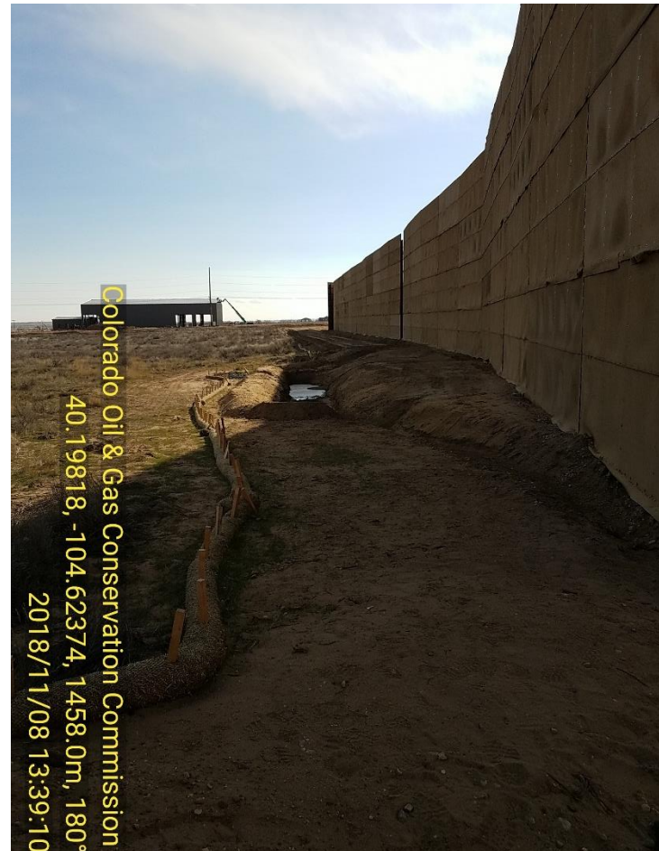
Photo 2 Storm Water BMP's East Side of Location
