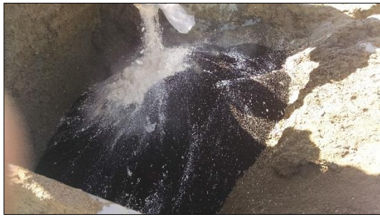
Mixing COGAC™ in Track Hoe Bucket
