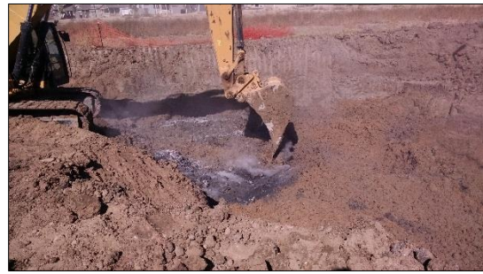
Mixing COGAC™ into Excavation with Track Hoe
