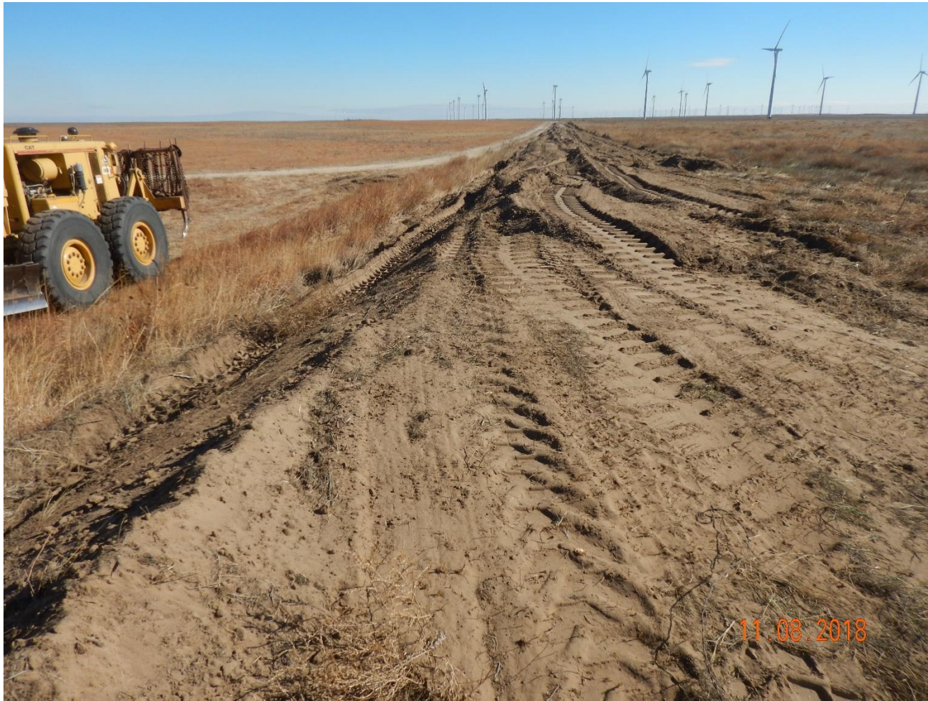
Photo 8: Photo taken from the north of the location. Photo shows a “wind blown” area where sediment deposition from the adjacent cropfield has built up over time. Operator is taking soils from this area to build up the pad and a portion of the access road that passes over a pipeline.
