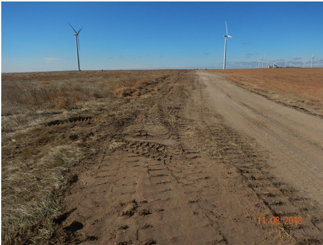
Photo 9: Photo taken from the section oil and gas access road that turns from North/south to east/west. Photo shows a “wind blown” area where sediment deposition from the adjacent cropfield has built up over time. Operator is taking soils from this area to build up the pad and a portion of the access road that passes over a pipeline.
