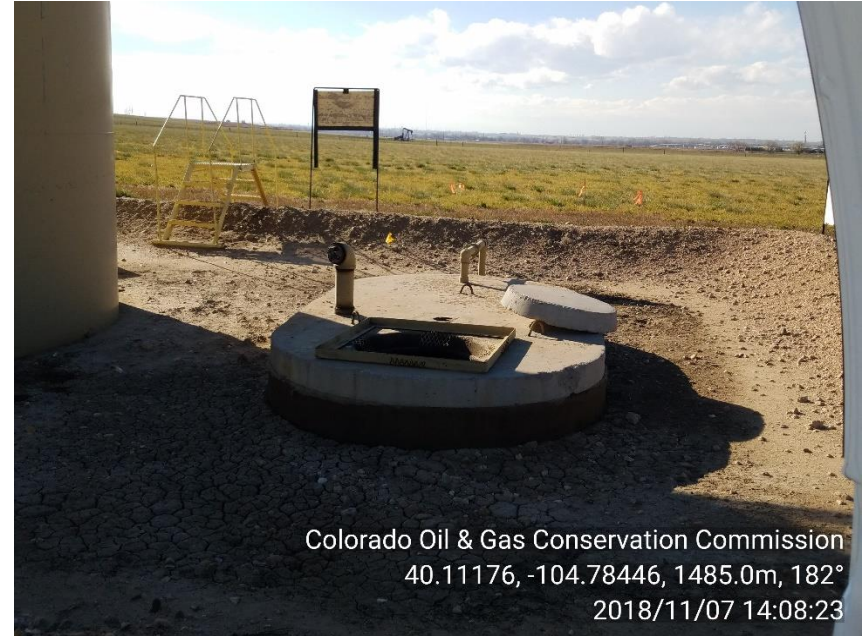
PHOTO 4: Lid to tank is removed and tank does not have any bird protection.
