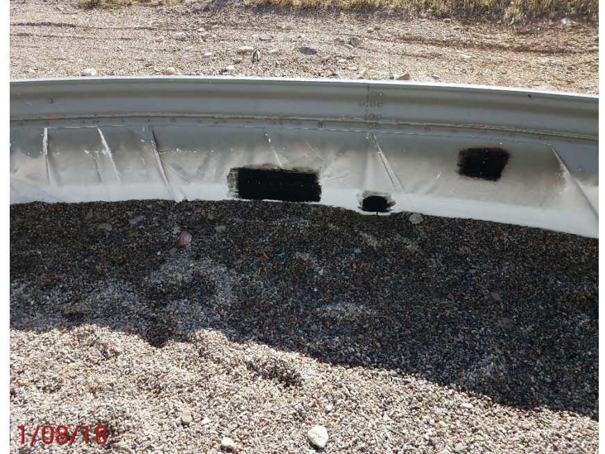
Location Photo #6, secondary containment repaired
