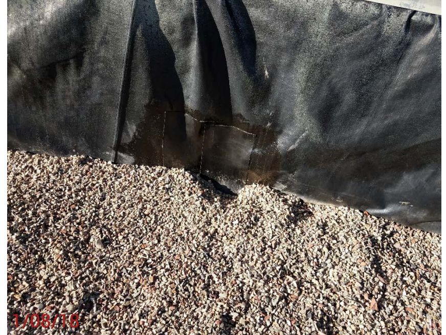
Location Photo #4, secondary liner repaired.
