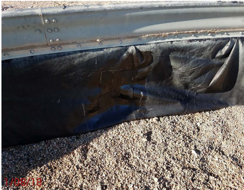
Location Photo #5, Secondary liner repaired
