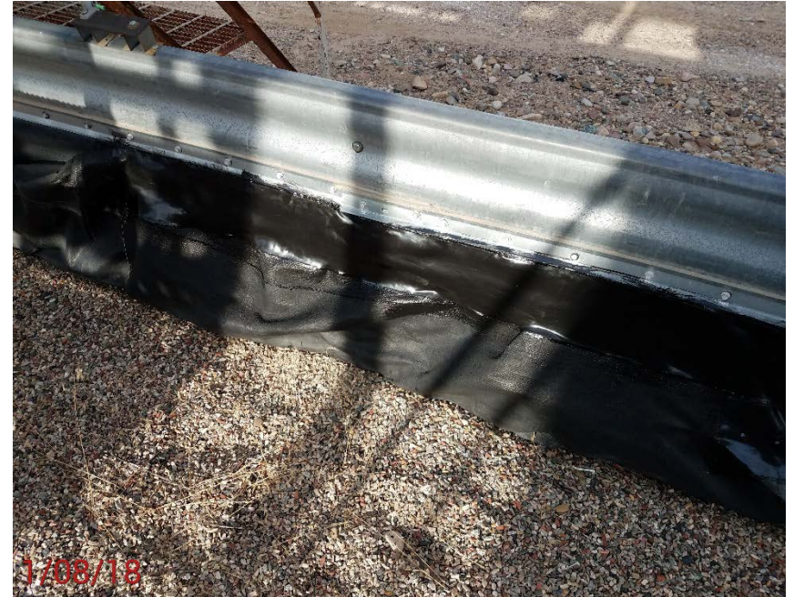
Location Photo #2, secondary battery containment repaired.
