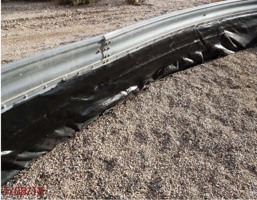
Location Photo #3, Secondary battery containment repaired.
