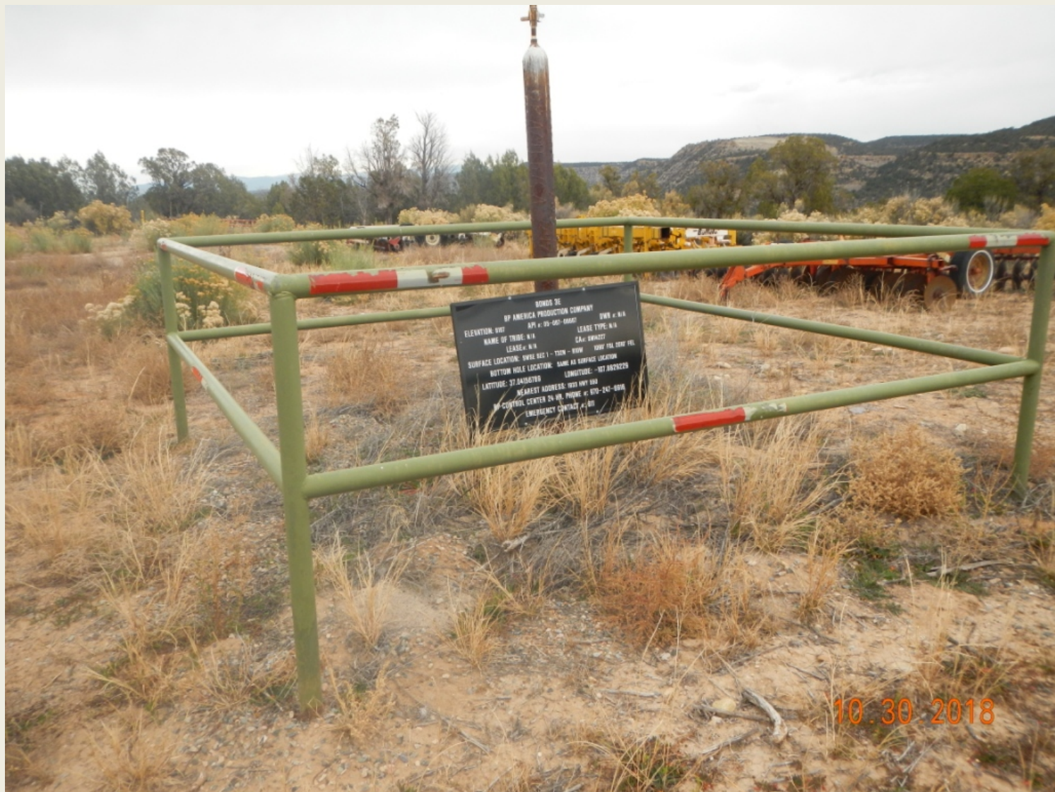
Photo 8. View of dry hole marker, barrier fencing, and signage at the plugged well head.
