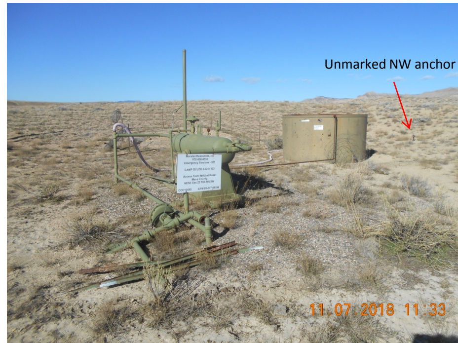
Separator with sign , blowdown pit, tank. Junk pipe, hose and valves. Unmarked NW anchor
