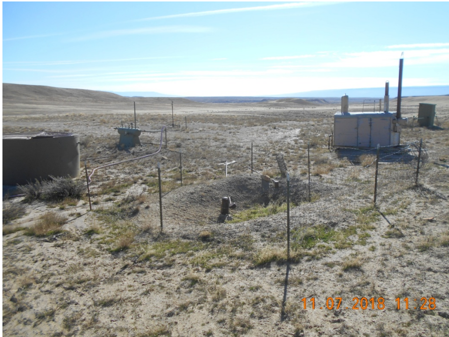
Overview of location from NW corner looking SE
