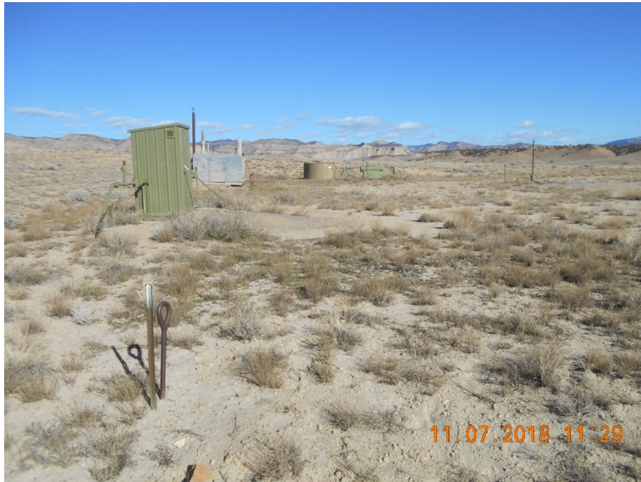
Meter housing and SW corner anchor with marker
