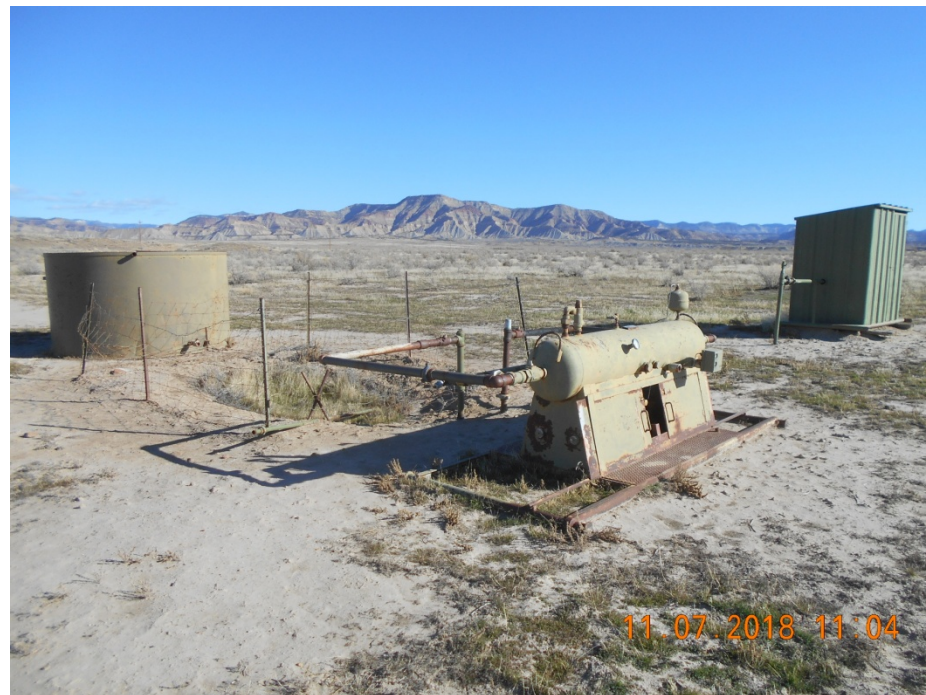
Separator , blowdown pit, tank and meter housing.
