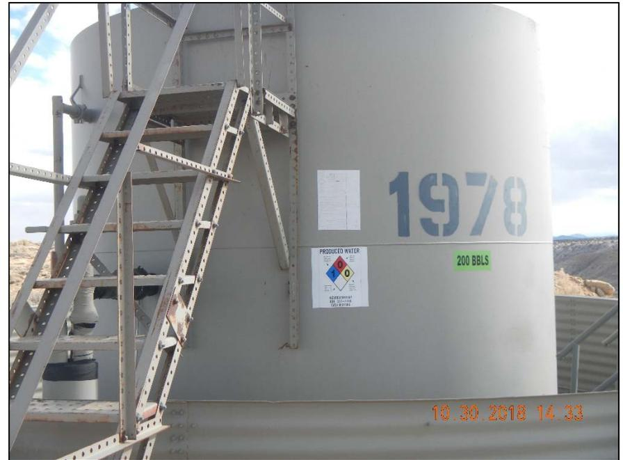
Photo 2. Produced water with NFPA flammability of "0".
