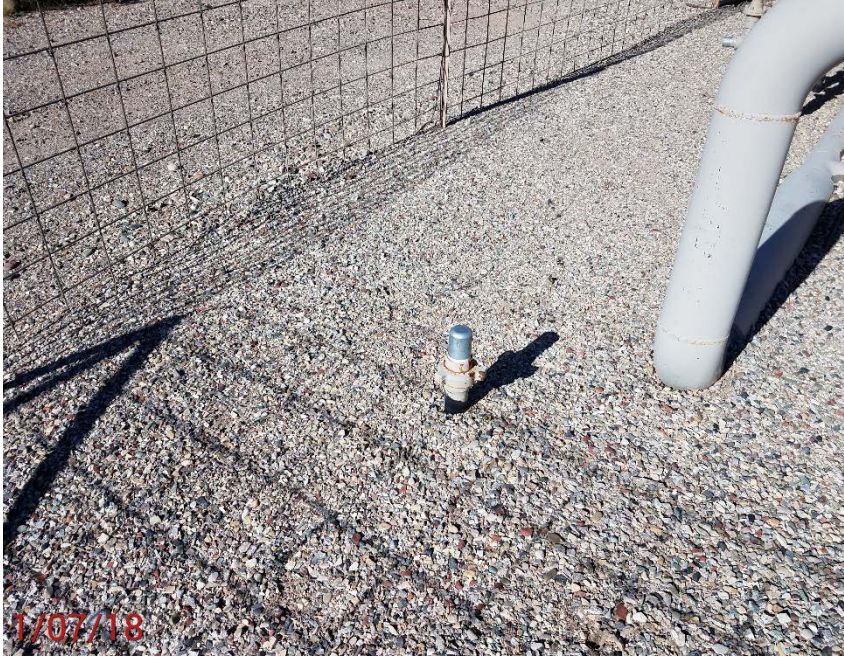
Location Photo #5, unmarked flow line riser, mark as required.
