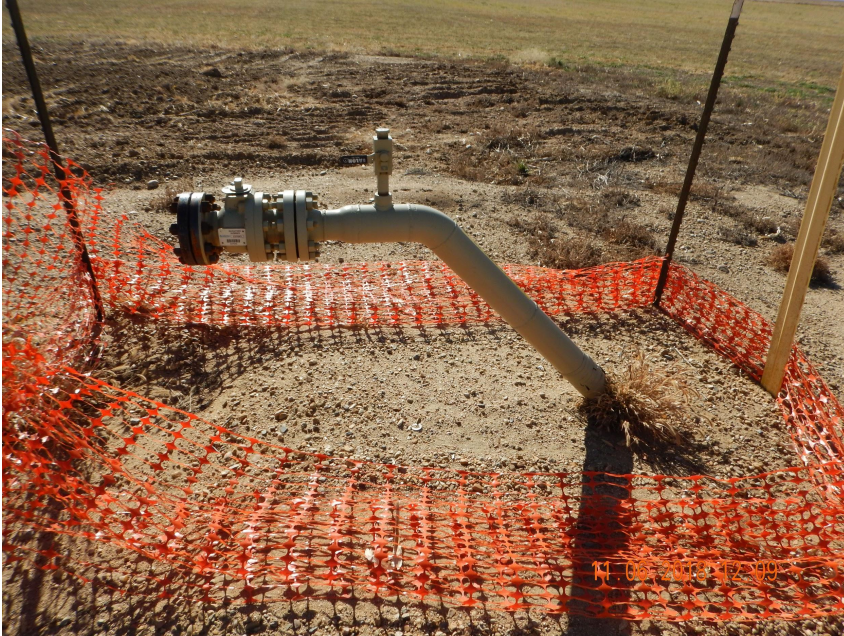
Photo 3. Photo taken from the tank battery location, facing South. Operator has failed to remove all equipment.
