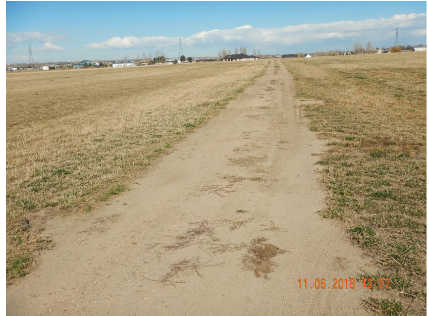
Photo 2. Photo taken from the entrance of the access to the location, facing North. Operator has failed to perform final reclamation activities (i.e., remove gravel, decompaction, seedbed prep and seed). Reference area vegetation is alfalfa (cropland).
