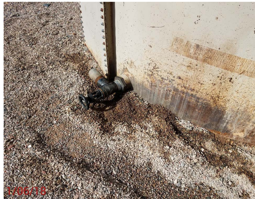
Location Photo #8, Oily stained rock in battery containment area.
