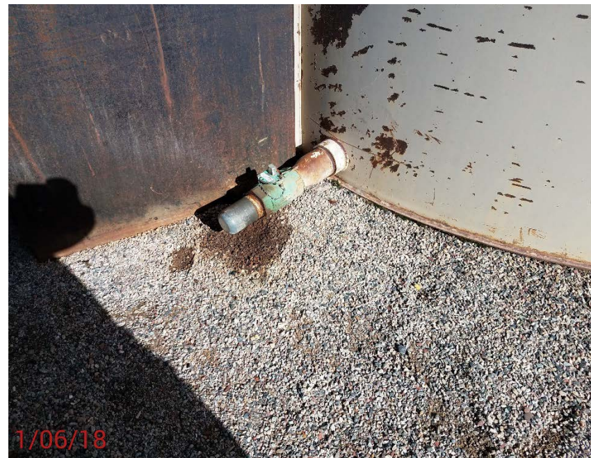
Location Photo #12, Oily stained rock in battery containment area.
