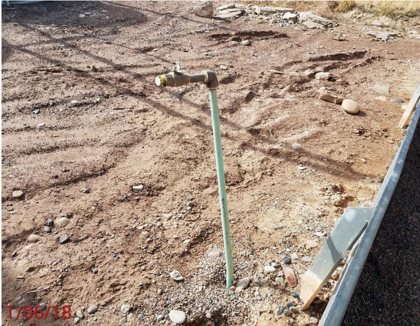
Location Photo #5, unmarked flow line riser.
