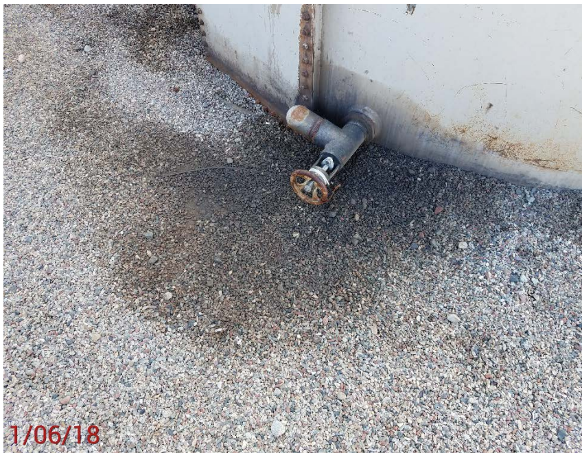
Location Photo #11, Oily stained rock in battery containment area.
