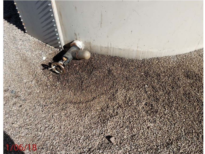
Location Photo #4, Oily stained rock in battery containment.
