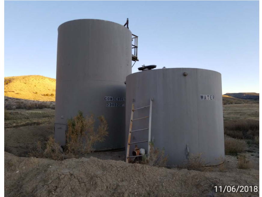
Tanks looking southeast
