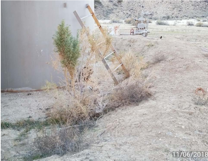
Weeds on berm and within berm area
