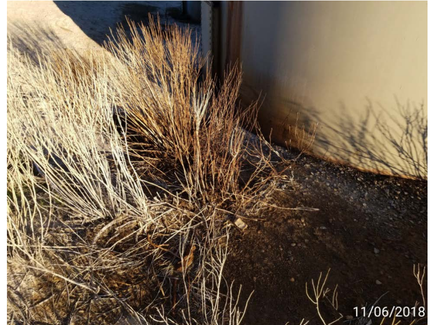
Condensate leaking from tank photo 3
