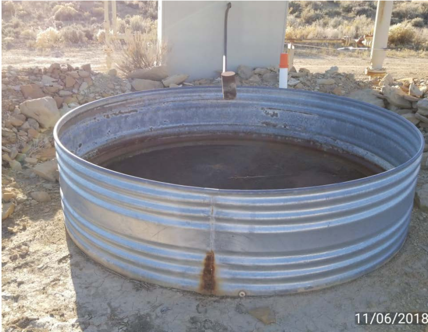
Tank with hole near bottom edge. Tank appears to be out of service.
