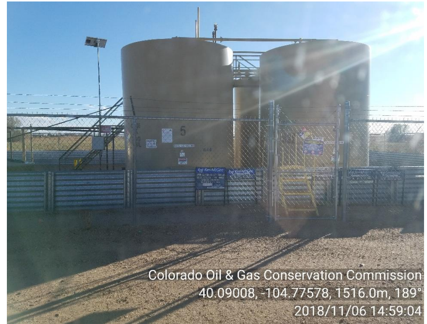
PHOTO 2: TANK BATTERY
