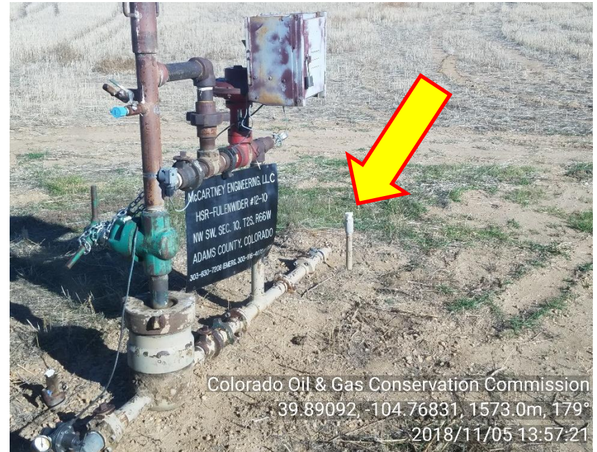
PHOTO 2: UNUSED EQUIPMENT/ CORRECTIVE ACTION REMOVE OR MARK UNUSED RISER
