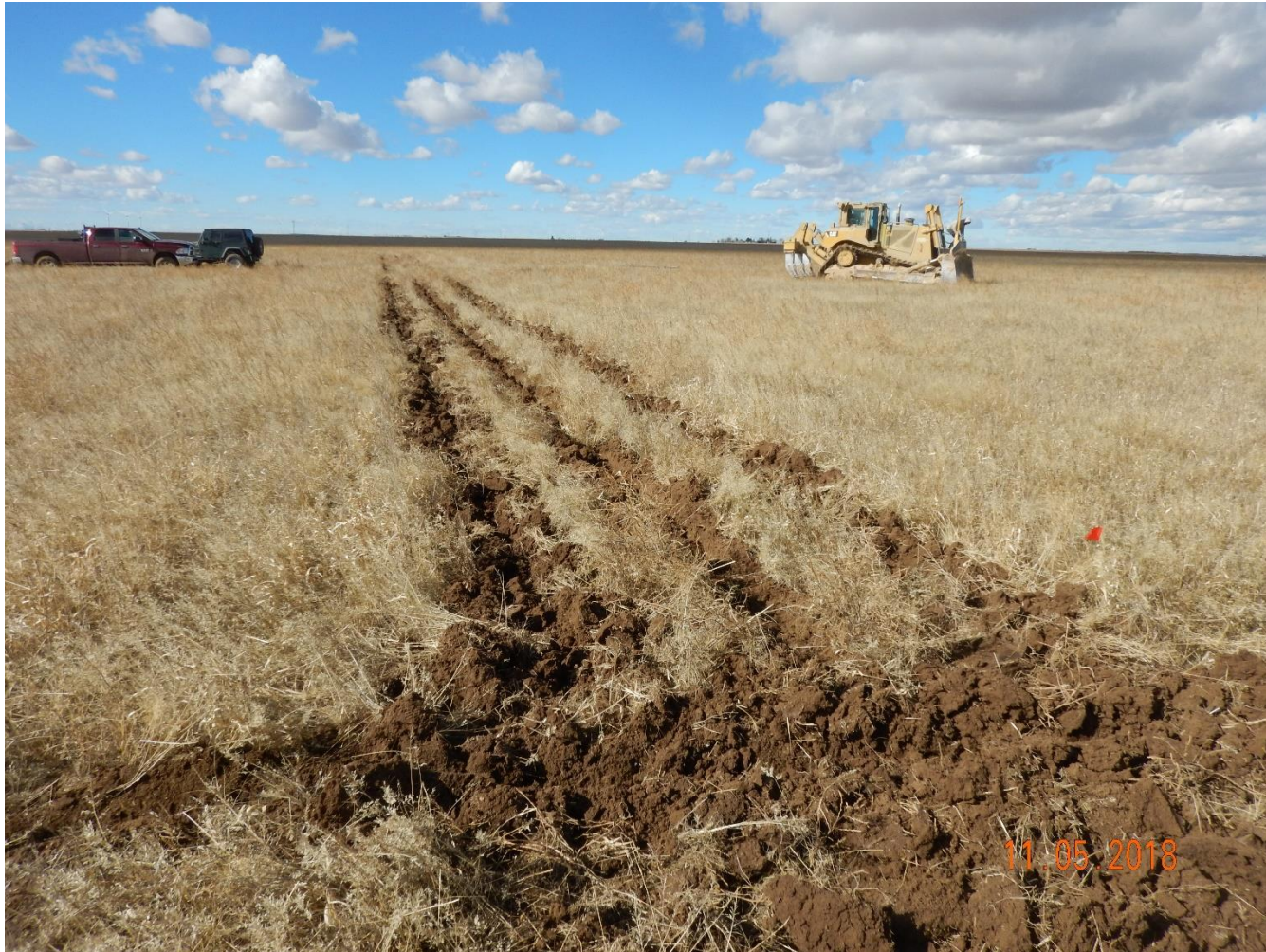
Photo 1: Photo taken from the southeast corner of the disturbance area, facing west. Photo shows construction in process. Photo also shows surface roughening has been used as a perimeter stormwater control
