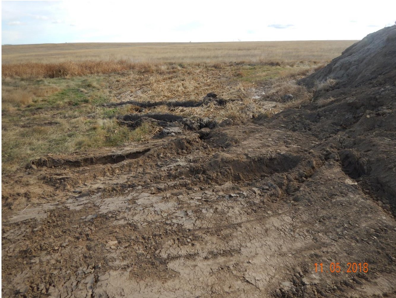
Photo 3: Photo taken from the northeast end of the pits, facing east. Photo shows area of the pit where water was discharging at the base. Spill appears to have been controlled.
