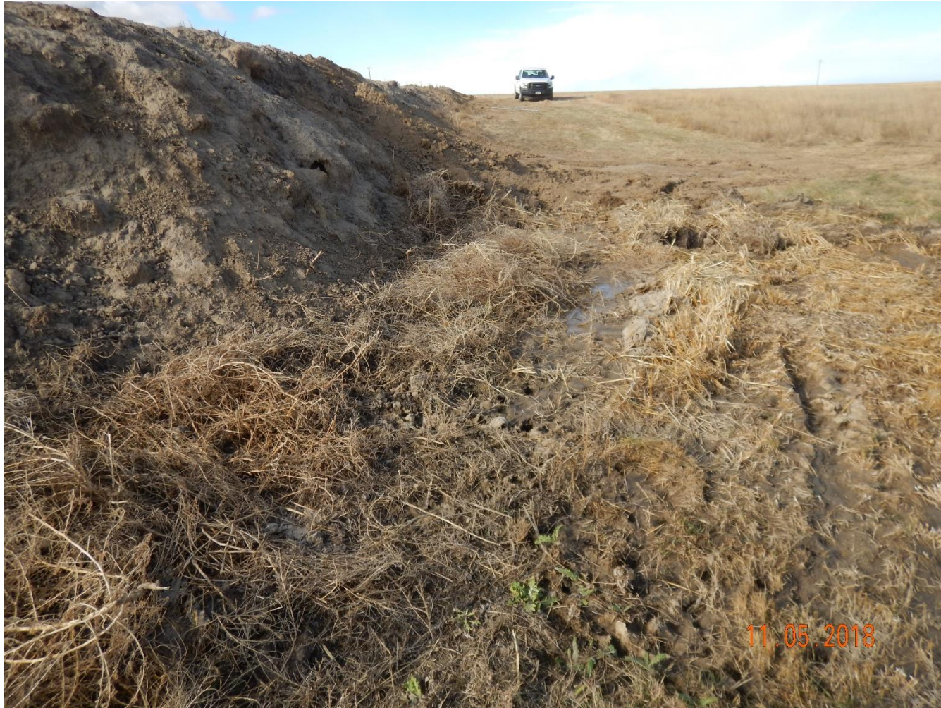
Photo 5: Photo taken from the northeast end of the pits, facing west. Photo shows area of the pit where water was discharging at the base. Spill appears to have been controlled, however, cleanup does not appear to have occurred.
