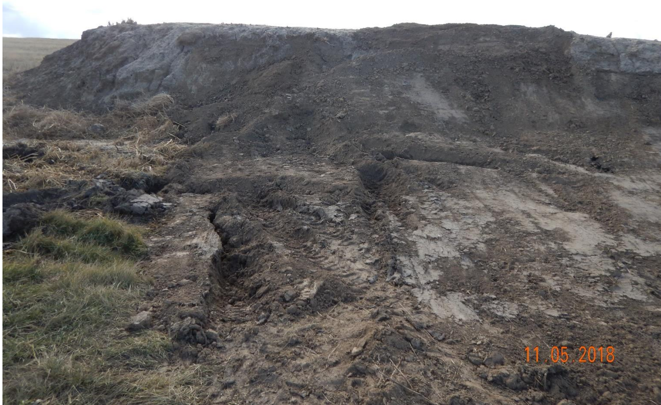
Photo 1: Photo taken from the northeast end of the pits, facing south. Photo shows area of the pit where water was discharging at the base. Spill appears to have been controlled.
