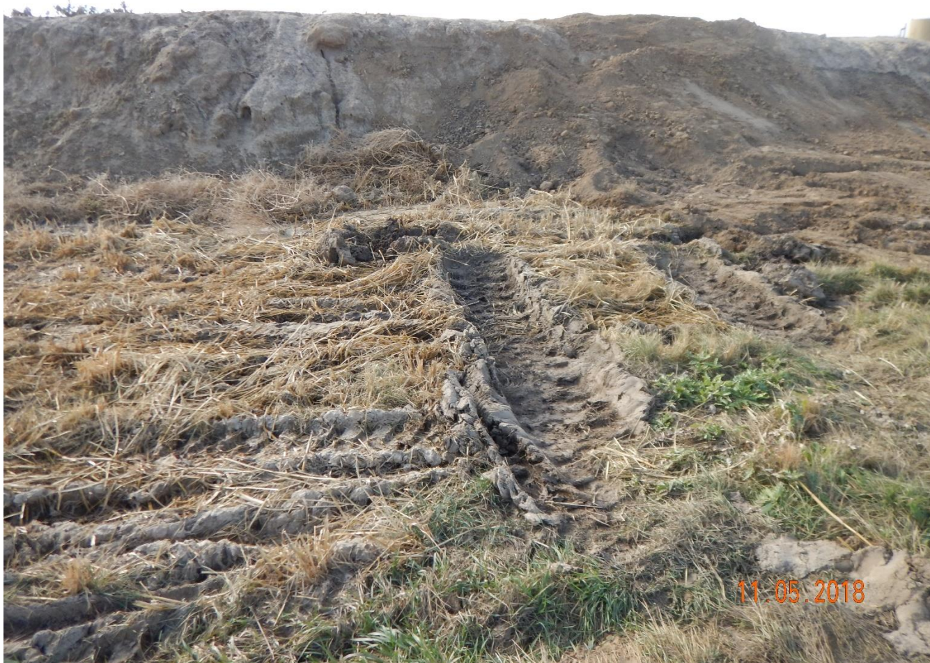
Photo 4: Photo taken from the northeast end of the pits, facing southwest. Photo shows area of the pit where water was discharging at the base. Spill appears to have been controlled.
