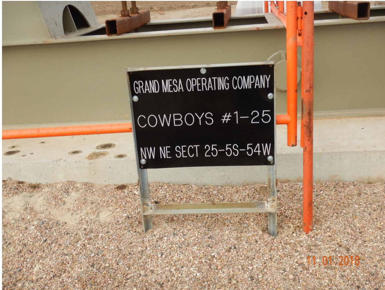
Photo 2: Photo taken from the east end of the pump unit. Photo shows sign. Sign at well missing operator contact/emergency number.
