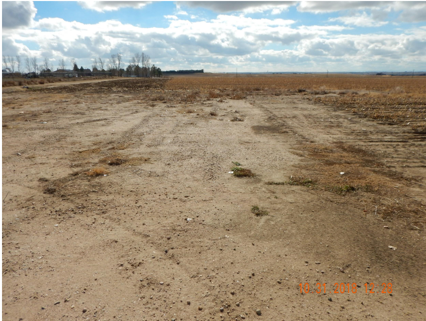
Photo 1. Photo taken from the central well and tank battery location, facing South. Operator has failed to perform final reclamation activities (i.e., remove gravel, decompact, seedbed prep and seed).
