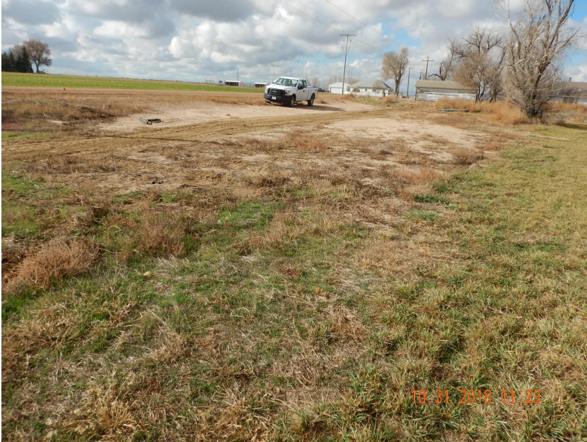
Photo 3. Photo taken from the eastern tank battery location, facing West. Operator has failed to perform final reclamation activities (i.e., remove gravel, decompact, seedbed prep and seed).
