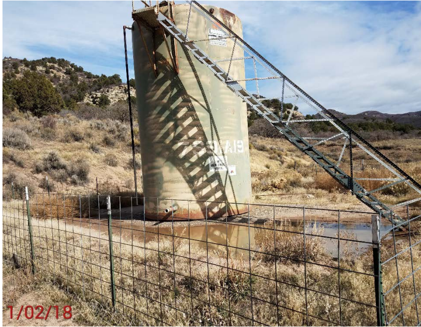
Location Photo #3 uncontrolled weeds
