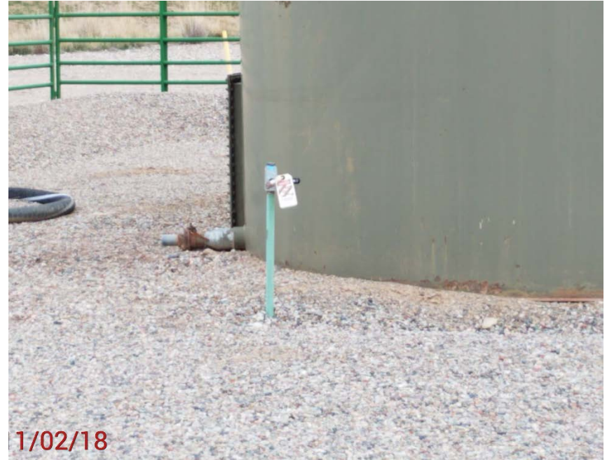
Location Photo #4, Flow line has been LO/TO
