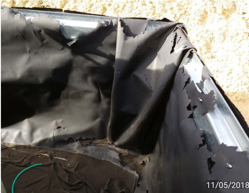
Tank liner on sides breaking apart.
