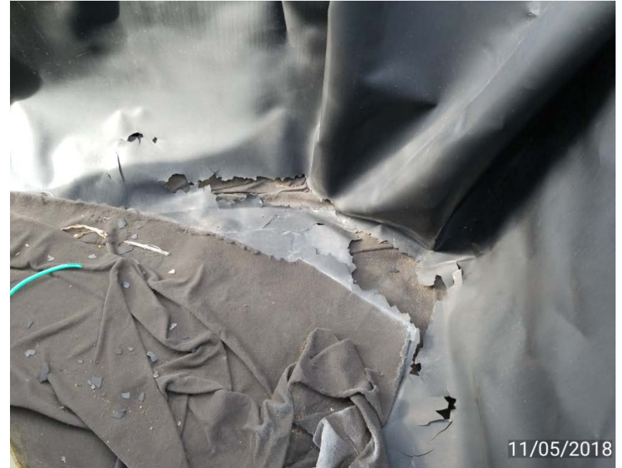
Tank liner at bottom breaking apart
