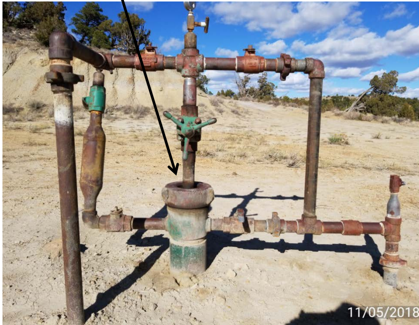
Gas leaking at well head – photo 1
