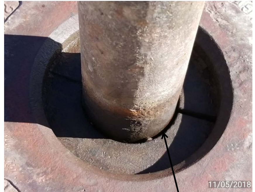
Gas leaking at well head – photo 2
