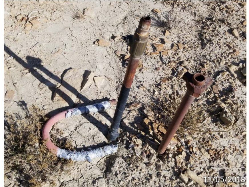
Uncapped risers next to meter building
