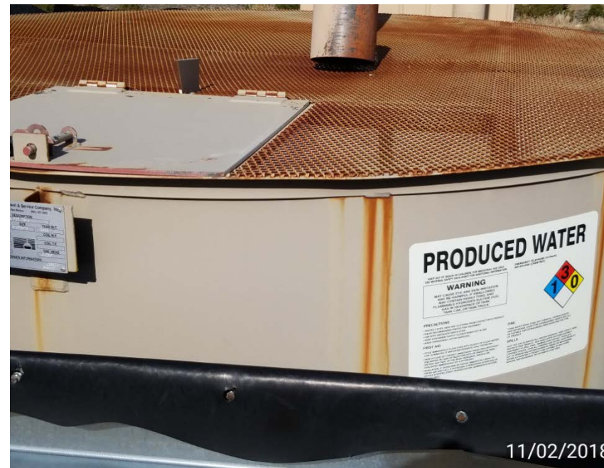
Tank missing capacity sign
