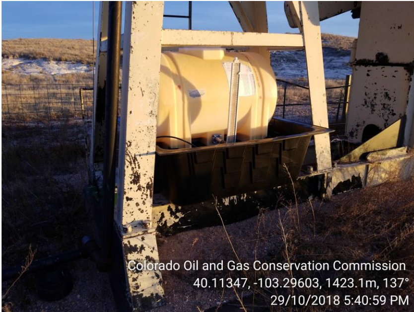
Photo 3: Chemical tank at wellhead.
