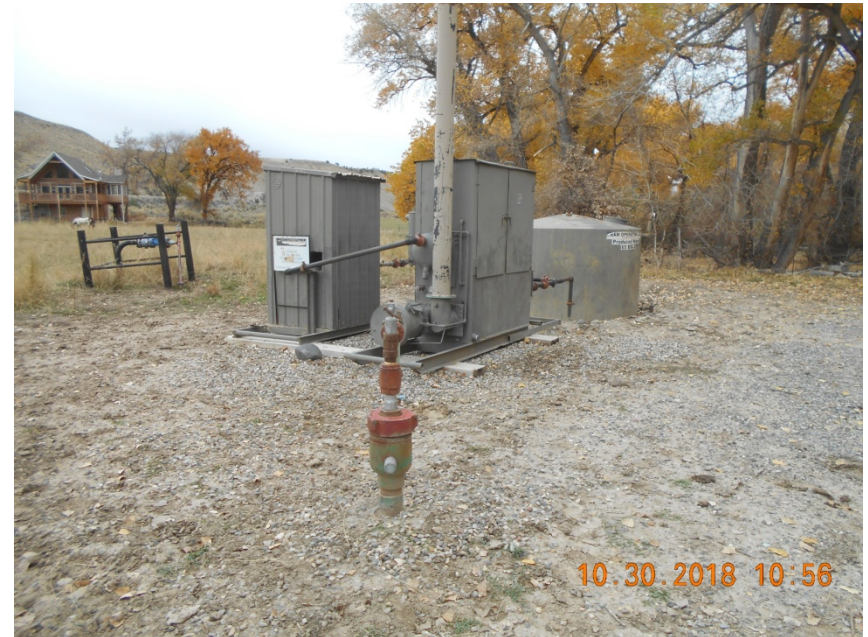
Location with Wellhead, Separator, Meter housing, Tank and flowline risers
