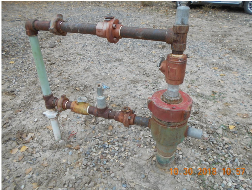
Wellhead with cut off surface casing exposed.
