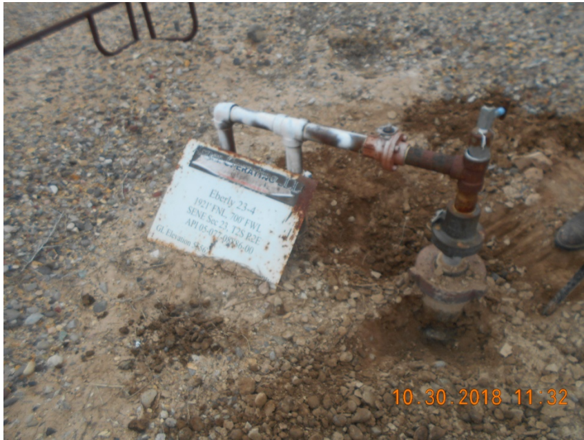
API # 05-077-08886 Eberly #23-4 Wellhead with cut off surface casing exposed.
