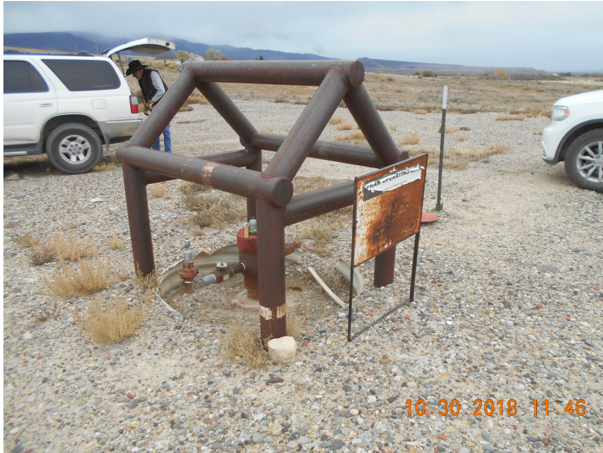
Wellhead with bradenhead valve exposed
