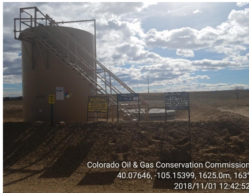
PHOTO 2: TANK BATTERY
