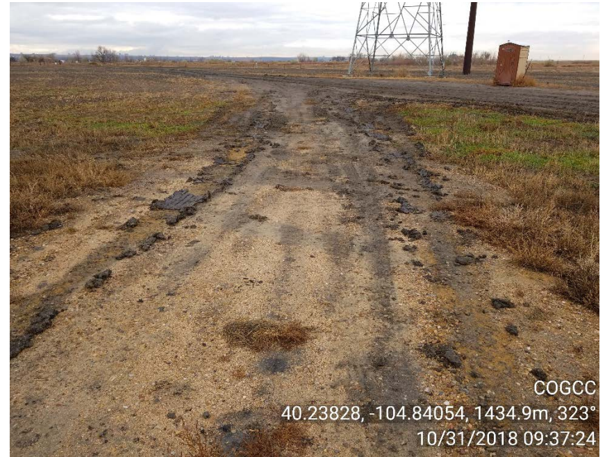
Photo 6 – Material being tracked of site
