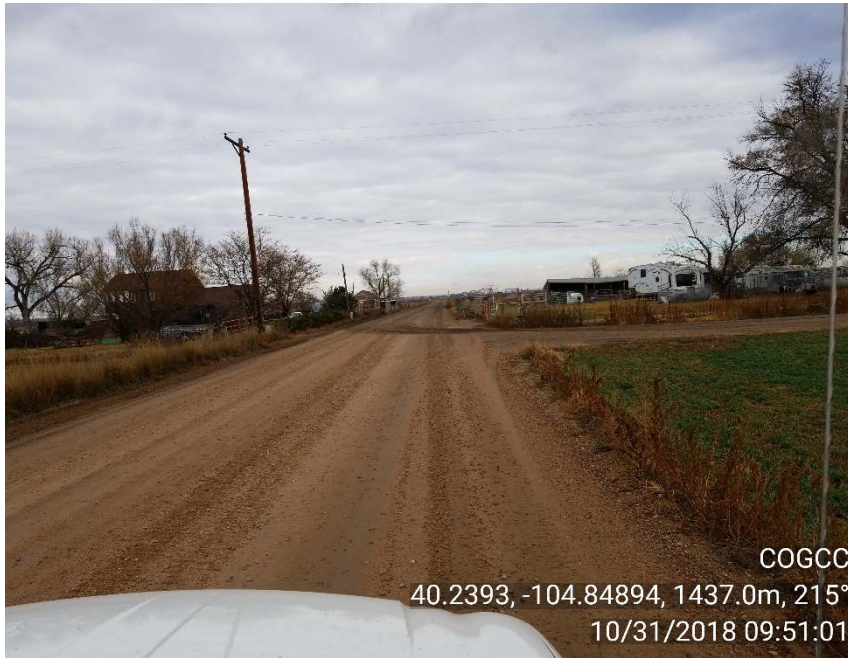
Photo 11 – Access road at county road
