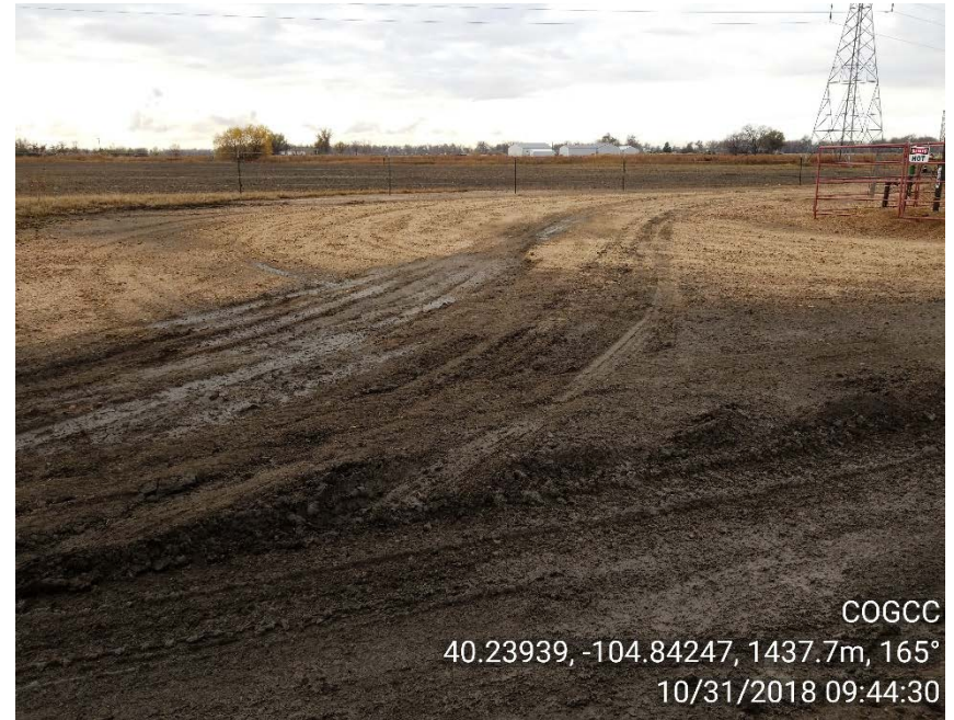
Photo 8 – Access road compared to nearby well site
