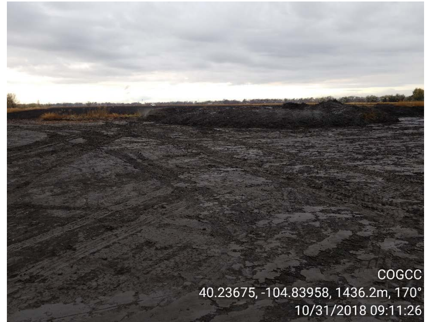
Photo 2 – Site Photo; Stockpiled material being spread at time of inspection
