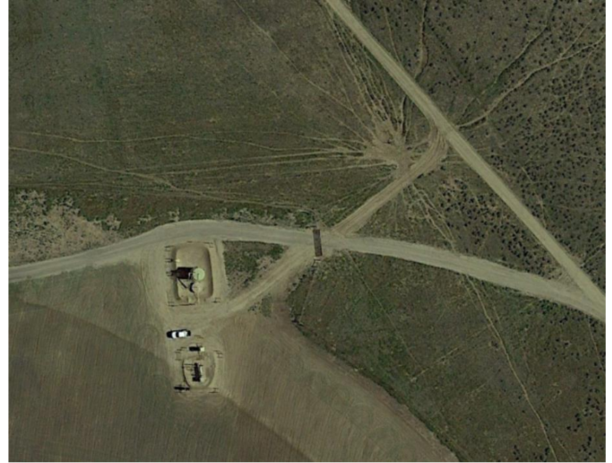
Access road during operations (5/31/2018)
