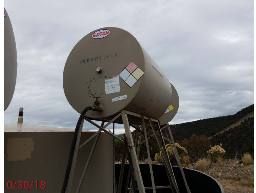
Location Photo #20, Missing labels on 500 gallon tanks.
