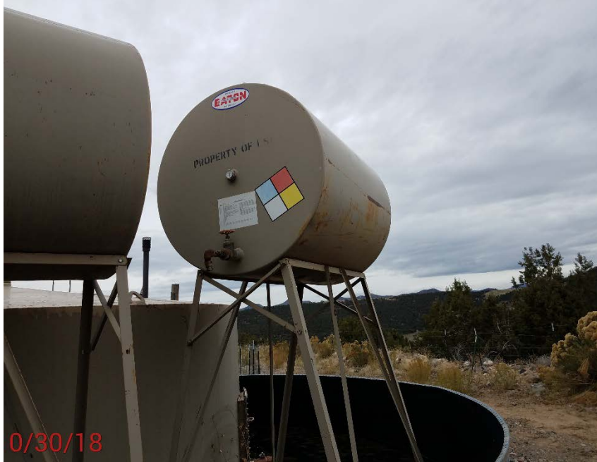
Location Photo #21, Missing labels on 500 gallon tanks.
