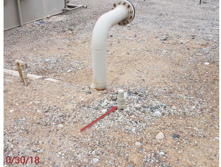
Location Photo #22, Unmarked flow line
