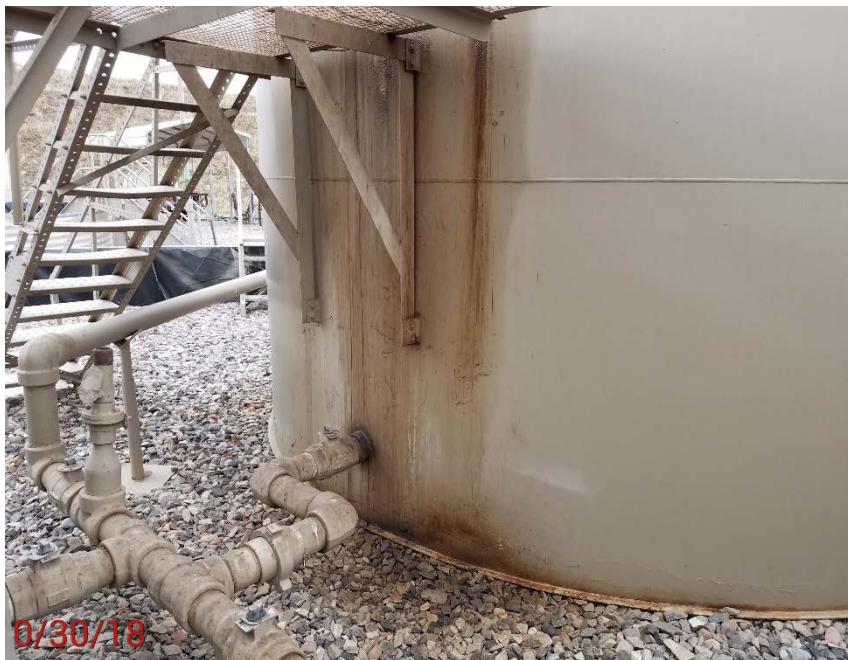
Location Photo #15, Mechanical condition of tank and valves
