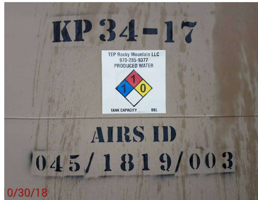
Location Photo #18, missing BBL capacity on all production tanks.
