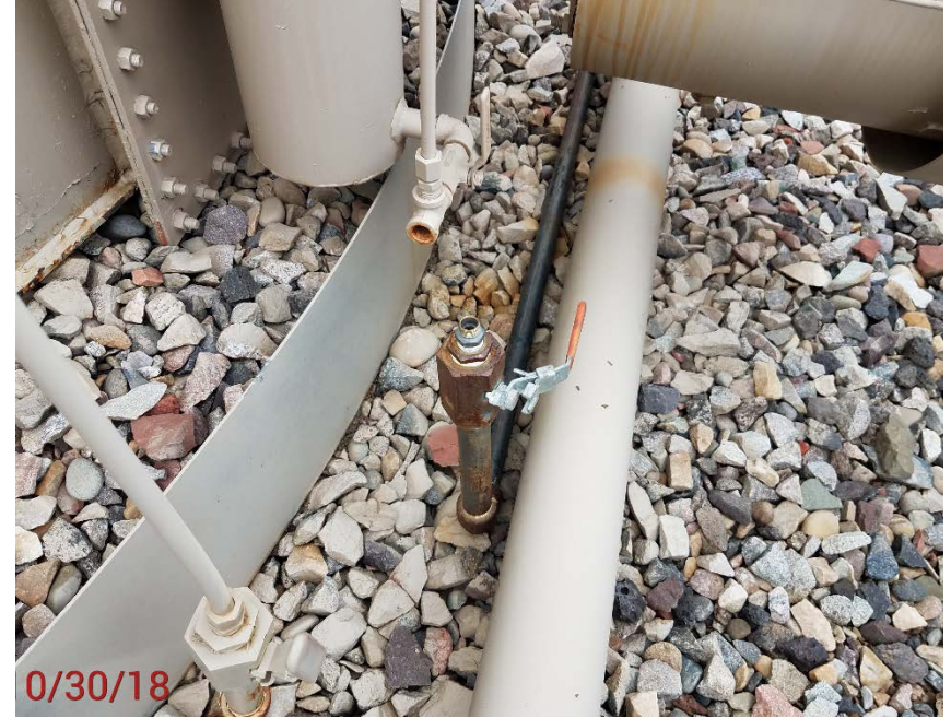
Location Photo #10, unused gas line in tank battery
