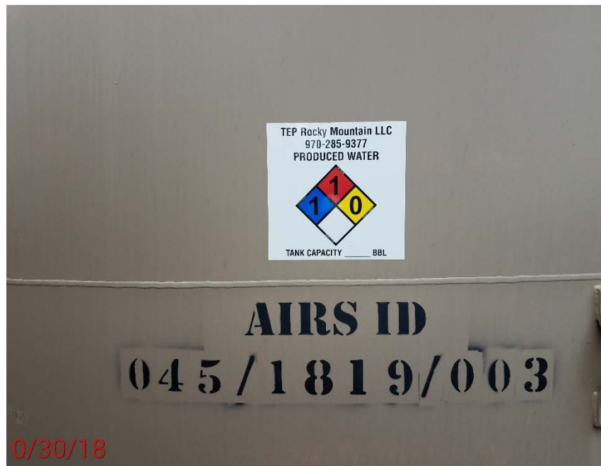
Location Photo #17, Missing BBL capacity on all production tanks.
