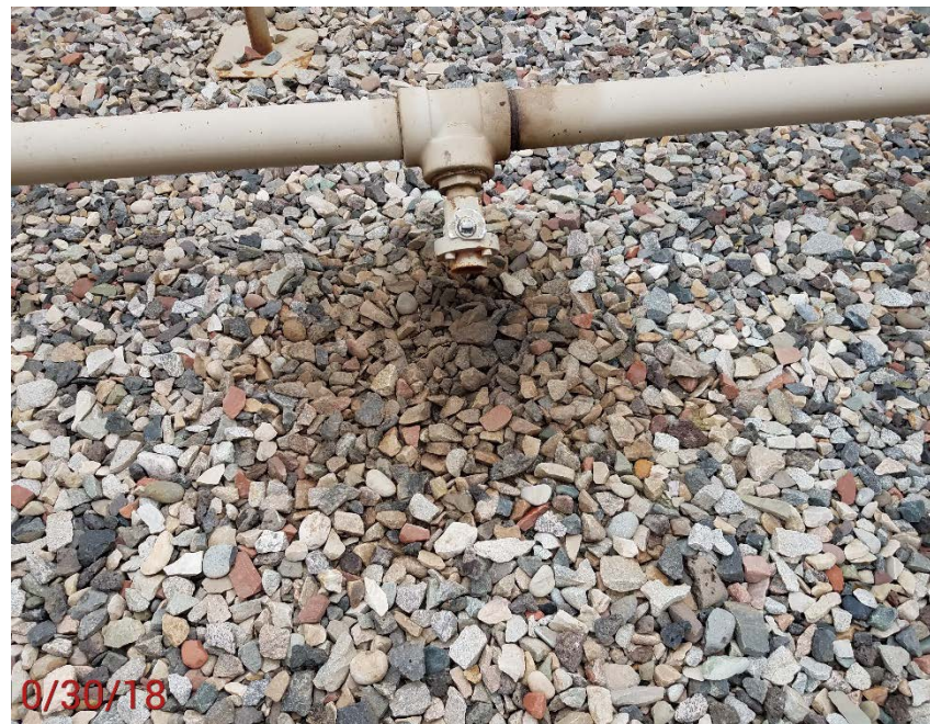
Location Photo #16, stained oily rock in battery containment.
