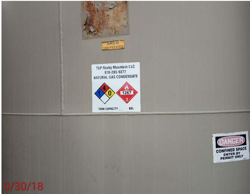
Location Photo #5, missing BBL capacity on all production tanks in the battery
