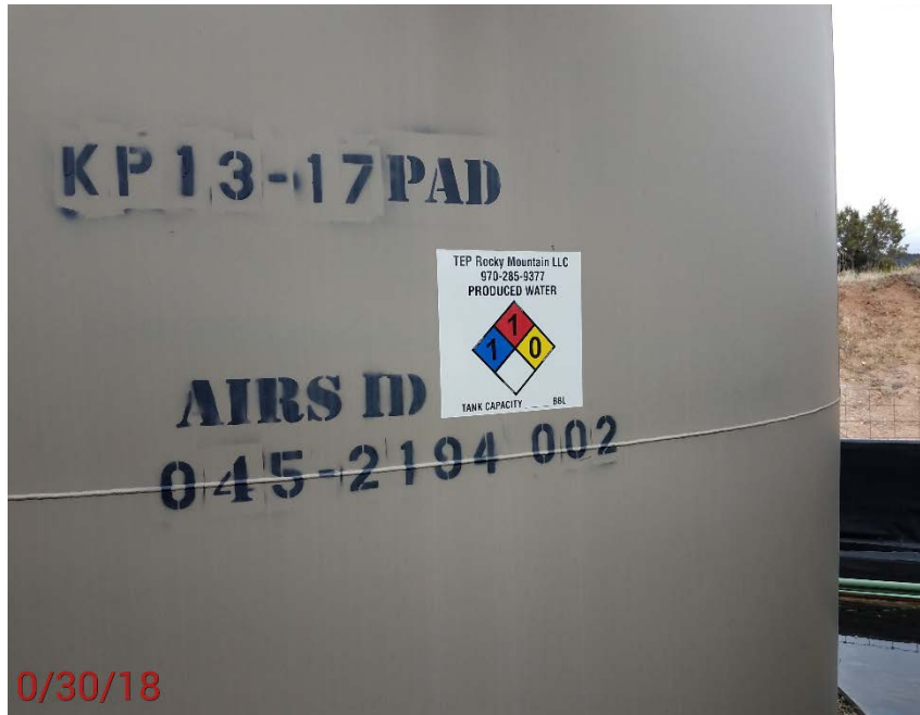
Location Photo #7, missing capacity on all tanks
