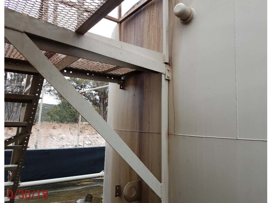
Location Photo #6, Oily residue down tank side
