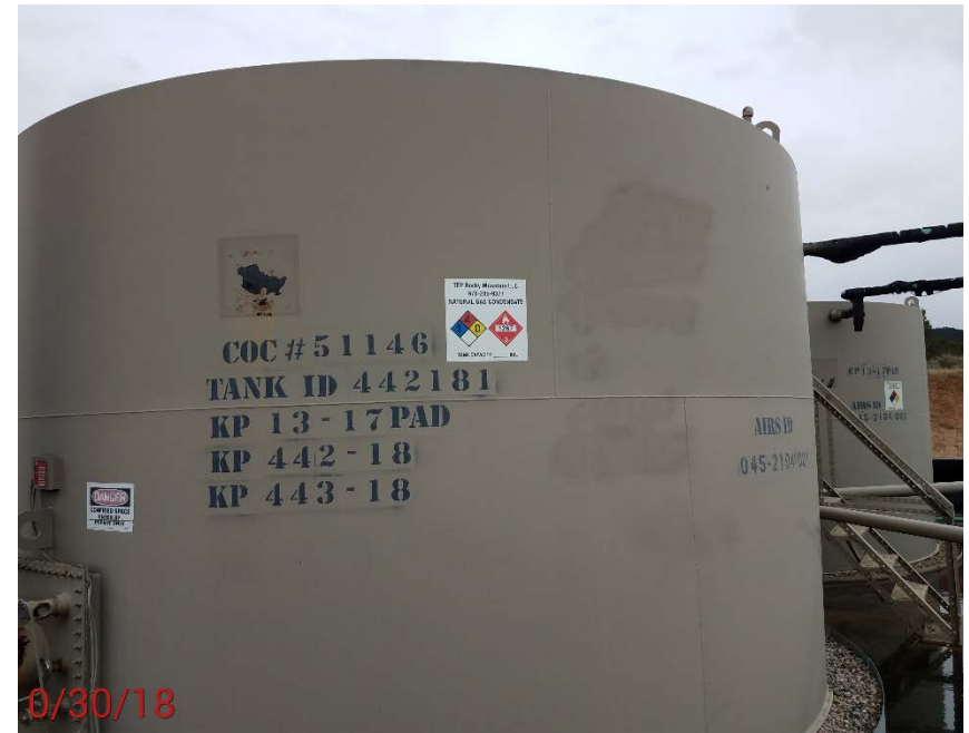
Location Photo #8, missing capacity on all tanks
