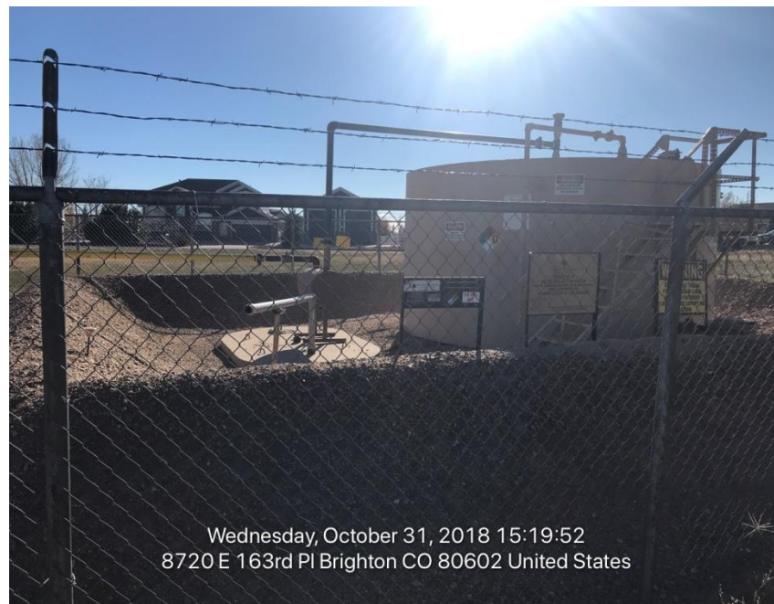
Photo#2 Production tank and produced water pit
